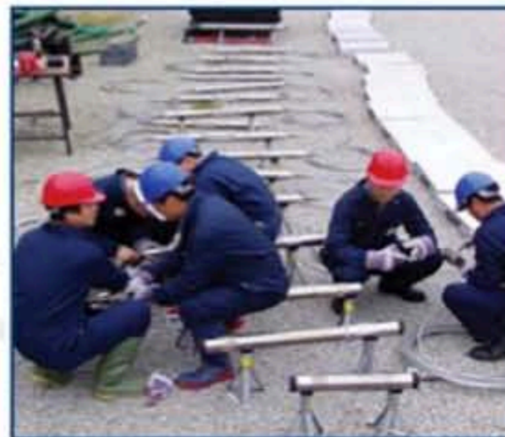
Commissioning a 16-level Geochain™ array
